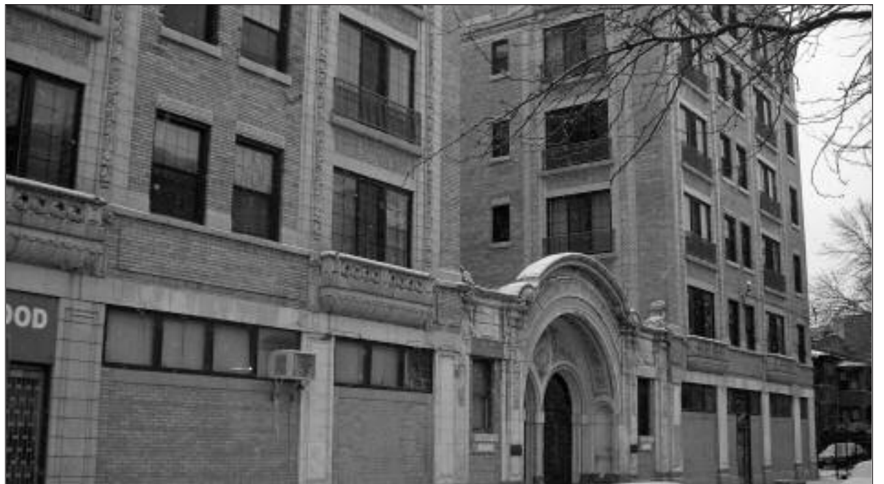
Conditions are improving for tenants of the Broadmoor Building (7600 N. Bosworth) with owner Lou Sopic undertaking extensive renovations of this Rogers Park landmark.
